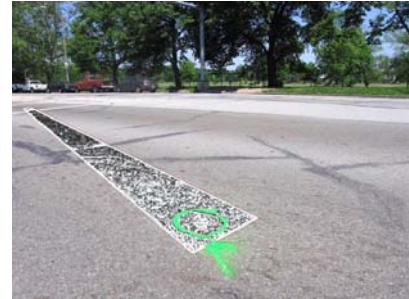
Location of axle under Skinker (looking NE towards Forest Park)
